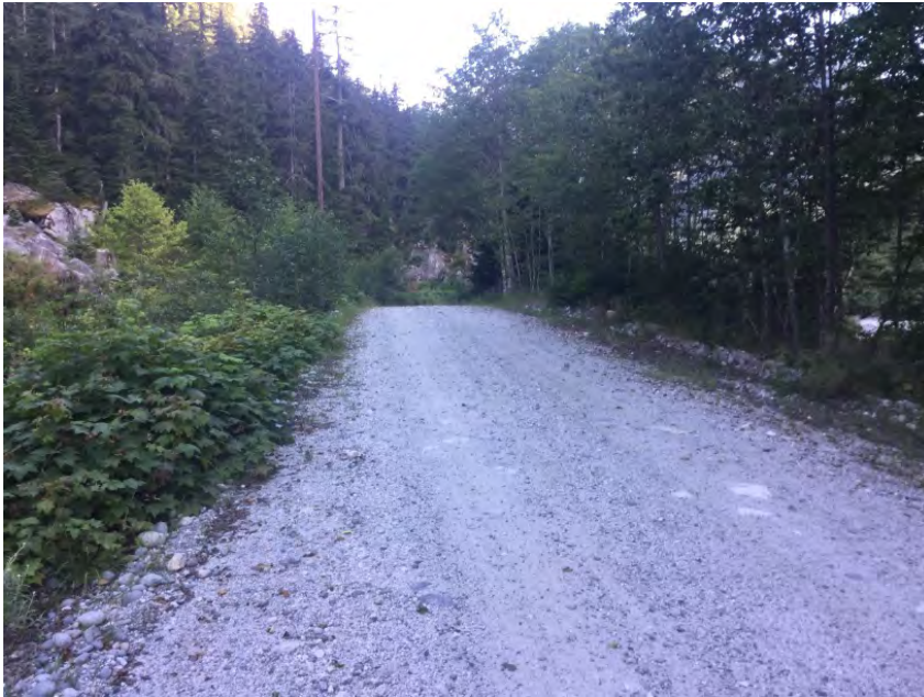
Right Approach Facing Towards Culvert
