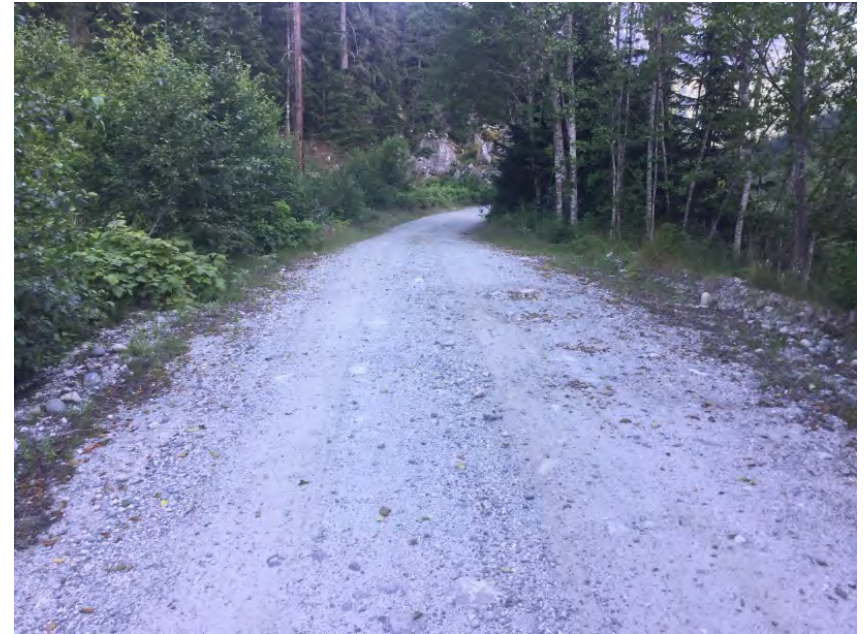
Roadway Over Culvert
