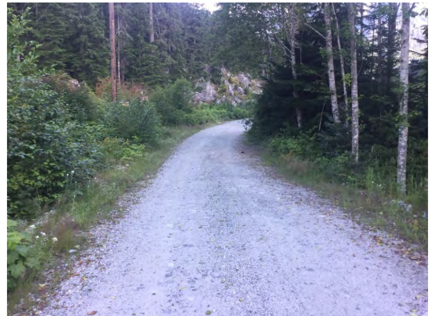
Left Approach Facing Away from Culvert
