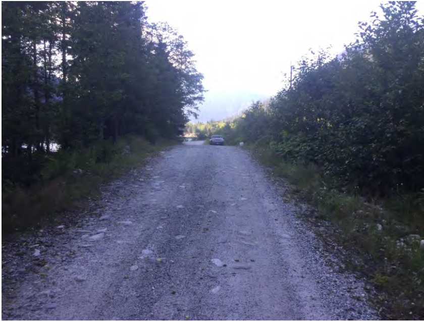
Left Approach Facing Towards Culvert
